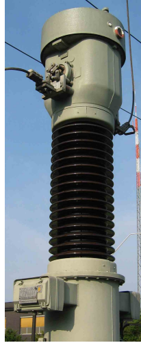
Figure 2.1: 110 kV Current transformer [45]
