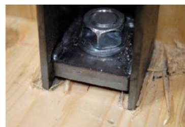
Wood crushing under hold-downs
