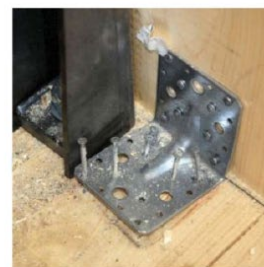
Nail withdrawal at angle brackets
