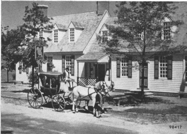
Fig. 7. Picture for which the percentage of "essential picture elements" has been measured. See p. 19.
