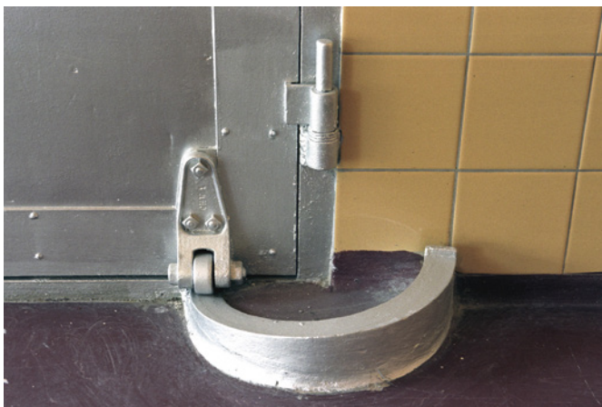
06 Example of the photographic documentation in the archive, showing the 'automatic' self-closing mechanism of a fire door. © Fas Keuzenkamp, 2007, coll. WDJArchitecten.
