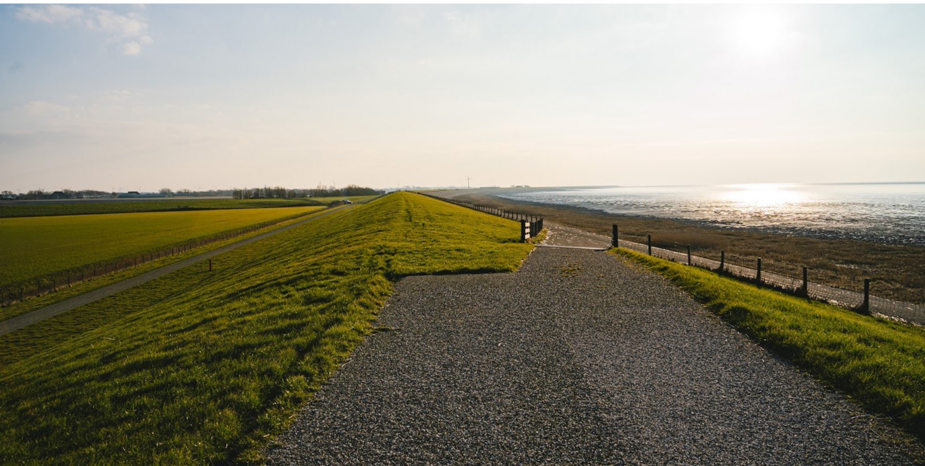
Sea dike segregation Photo: Author, 2022.
