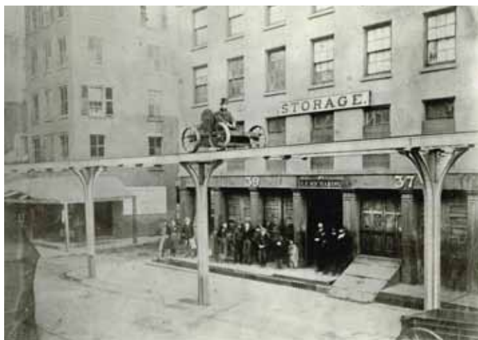
Figure 7.1.5. The West Side and Yonkers Patented Railway tested by Charles Harvey: December 1867
