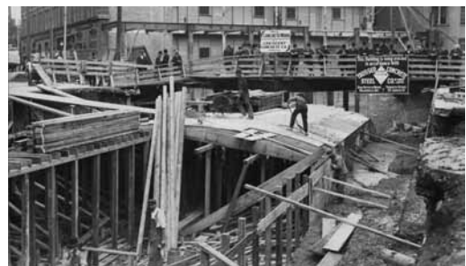
Figure 8.5.4b. Constructing an Eaton Subway under Albert Street for Eaton's, c.1912
