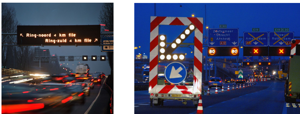
(a) Dynamic Route Information Panel (DRIP) on motorway A13 (©Rijkswaterstaat) (b) Work zone and active MTM system on motorway A1
