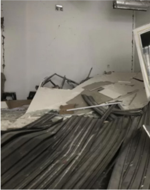
Photograph of damages in Marfa Gallery due to the August 4 explosion.
