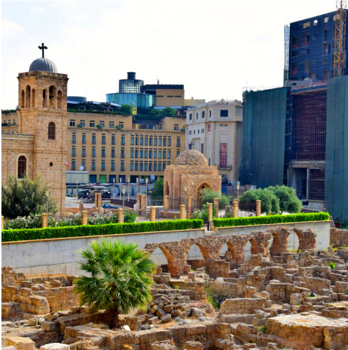
ongoing demolition & re-construction
