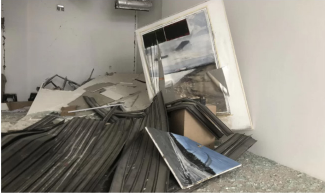
Photograph of damages in Marfa Gallery due to the August 4 explosion. Image courtesy of Marfa Gallery.
