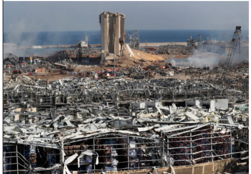
Workers and security officers work at the scene of an explosion that hit the seaport of Beirut, Lebanon, Wednesday, August 4, 2020. Photo courtesy of AP Photo/Hussein Malla.
