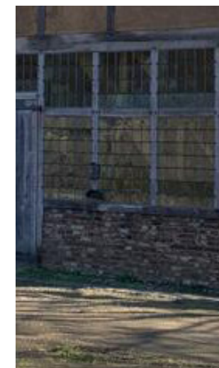
First meter of bricks & stained glass
