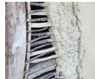
loam mixture is put on the wall
