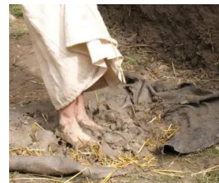
mixing of loam with straw
