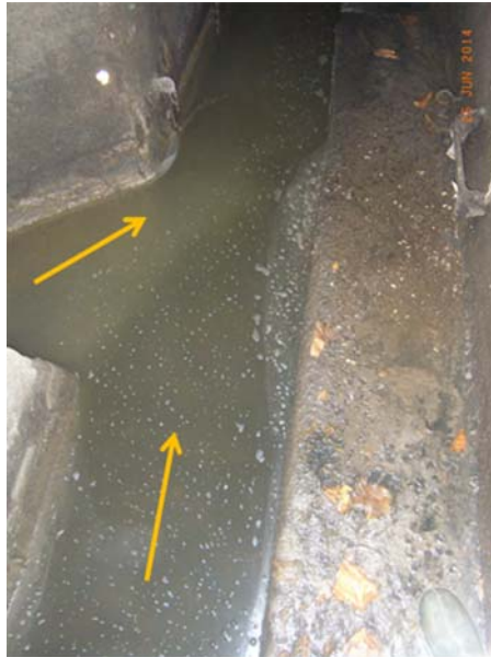
Figure 3.7 The water flowing from the left side channel influences the flow coming from the bottom. Source: Université Gustave Eiffel.
