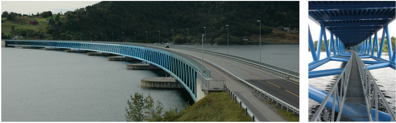
Figure 1: Left: The Bergsøysund Bridge viewed from the north end; right: the truss structure as viewed from below the bridge deck. Photo: K.A. Kvåle.
