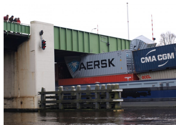
(b) Collision with the bridge 'Burgumersdam' on the Dutch canal 'Prinses Margriet'. The vessel involved was the CEMT Va class 'Fides' carrying 114 empty containers. [De Boer, 2011] [Brolsma, 2013]
