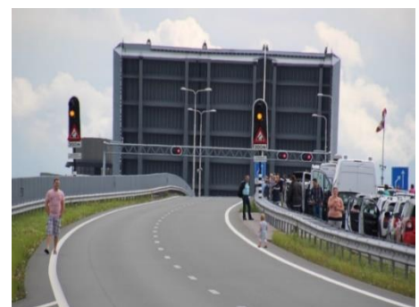
Figure 3. Malfunctioning movable bridge
