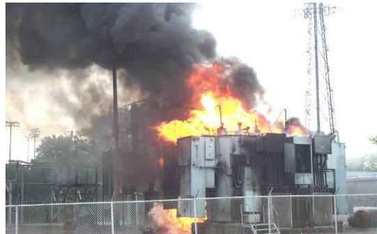
Figure 2.1: Transformer that failed [4].
