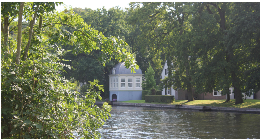
Figure 4. Country houses and estates were constructed next to the river Vecht as part of Holland's seventeenth century recreational landscape. Townhouses were built closely to the river side (source: G. Verschuure-Stuip, 2011)
