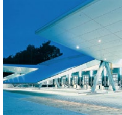
Ernsting Distribution Depot, Schilling Architekten
