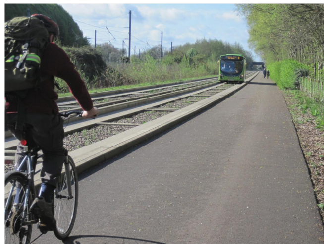
Fig. 1. The Cambridgeshire guided busway.
