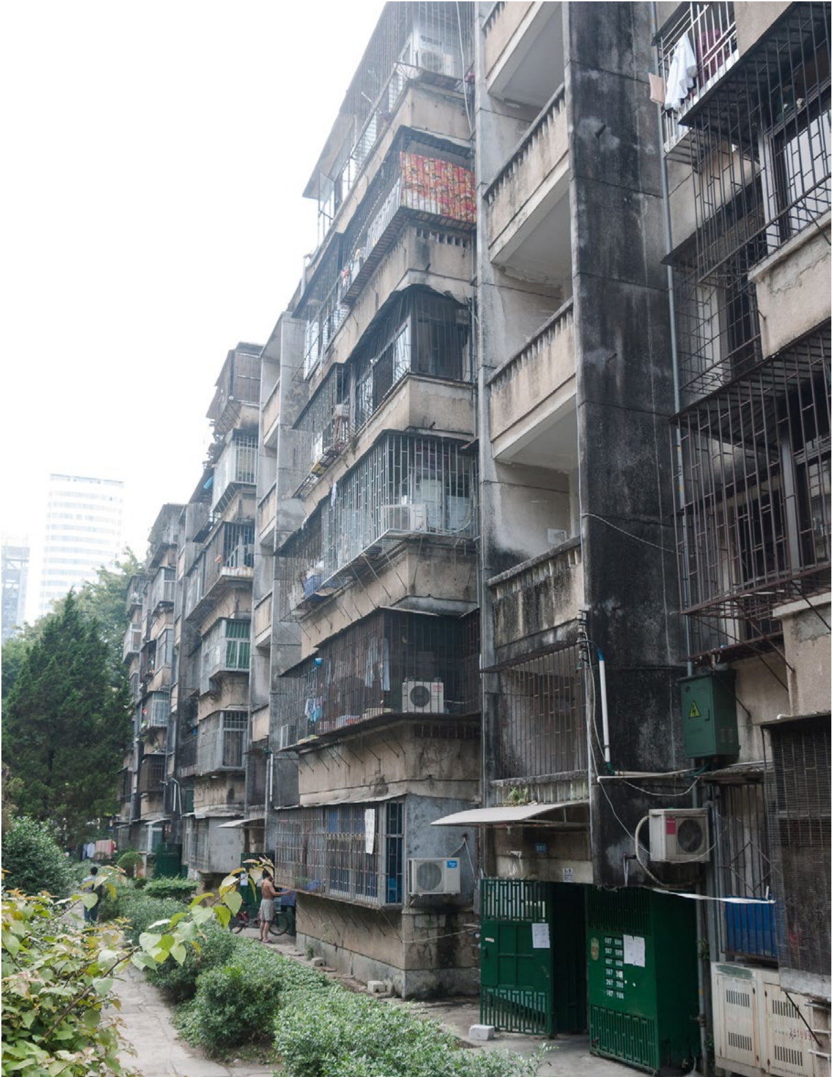
Residential building (Photo by author)
