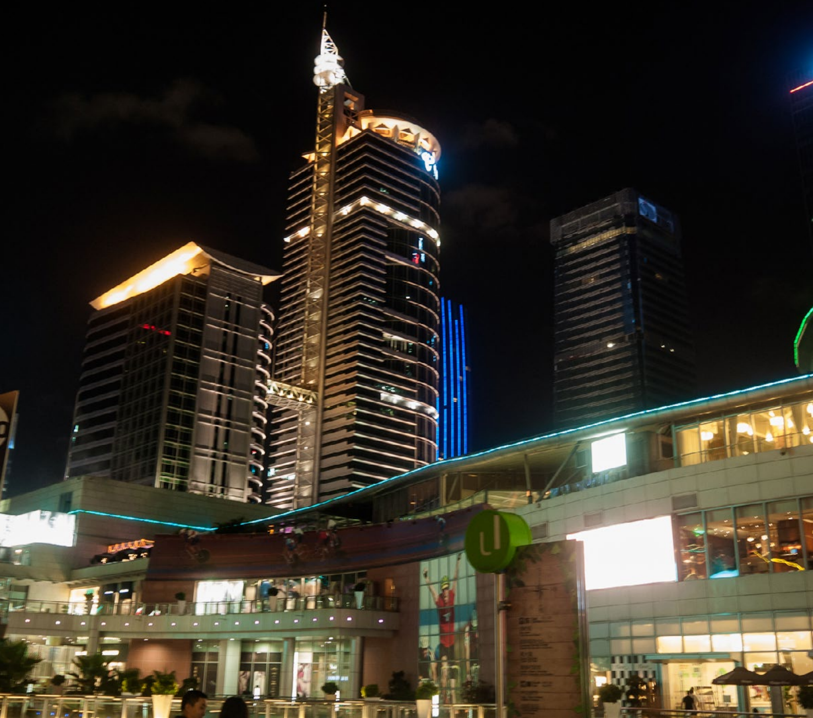
Development focuses on high-end shopping malls, offices and housing, which are unaffordable for low-income group (photo by author)
