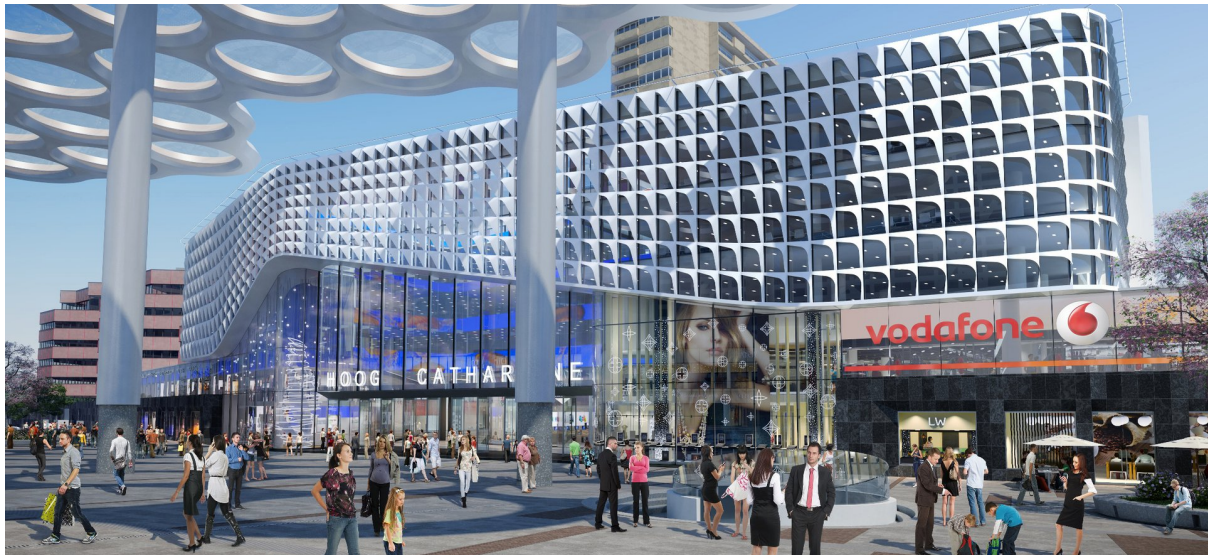
Figure 28: VodafoneZiggo's Central Office opposite Utrecht Central Station (VodafoneZiggo, 2017b)
