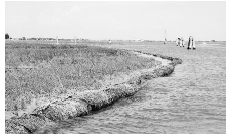
03 fig. 07/07 From top to bottom. The growth of an artificial barena: after 12 (01), 24 (02), and 36 (03) months. Vegetation and sediment accumulated will incorporate slowly the borders.
