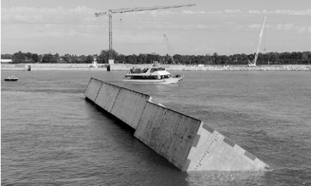
fig. 03/09 Mo.S.E. movable sluices during a test in Lido inlet. Source: mosevenezia.eu
