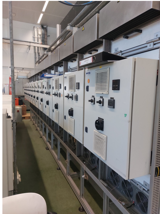
Figure 3.1: Light soaking machines at HyET which were used for light soaking the modules at OC and SC conditions
