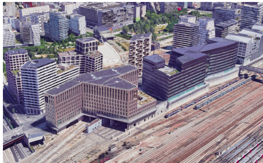
Existing over track development in Paris Clichy-Batignolles. Source: Google Earth
