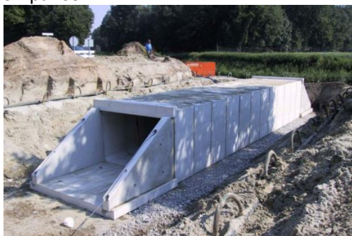
Figure 63 Applied culvert: Koppelduiker R2 (Romein, 2018)
