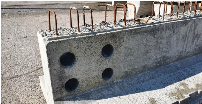
Figure 22 Haitsma concrete girder with extended stirrups
