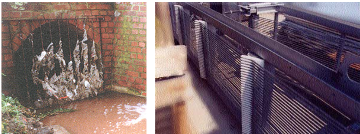
Figure 2-3: On the left an end of pipe bar screen (Water-Technology) and on the right a horizontal CSO screen (Headworks® Inc.)
