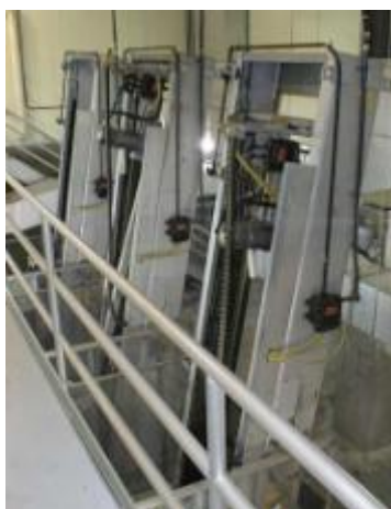
Figure 2-5: Inclined bar screen (Lenntech Water treatment & air purification Holding B.V.)
