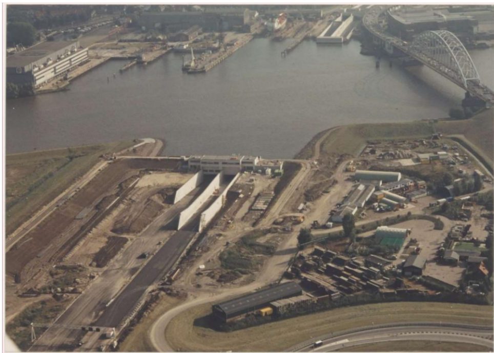
Figure 1.1: The Noordtunnel under construction (SWECO, 2020)
