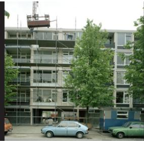
1984 First renovation (wooden frames replaced by plastic)
