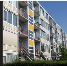
Current situation: red balconies and doors; white grid; yellow staircases; parapets with different colors; sunshade, paintwork in poor condition
