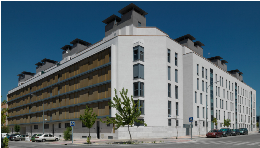
—> Figure 6.12: In this picture, big extruded stack ventilation chimneys from the roof can be seen. Source: feilden Clegg Bradley studio, n.d.
