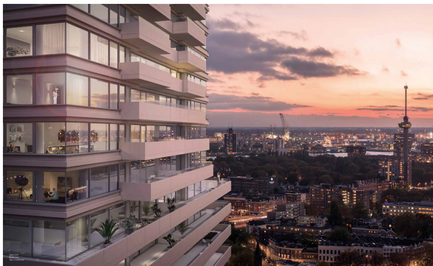
—> Figure 7.4: Continuous ribbon balconies shade mid-crown apartments. Source: V8 architects
