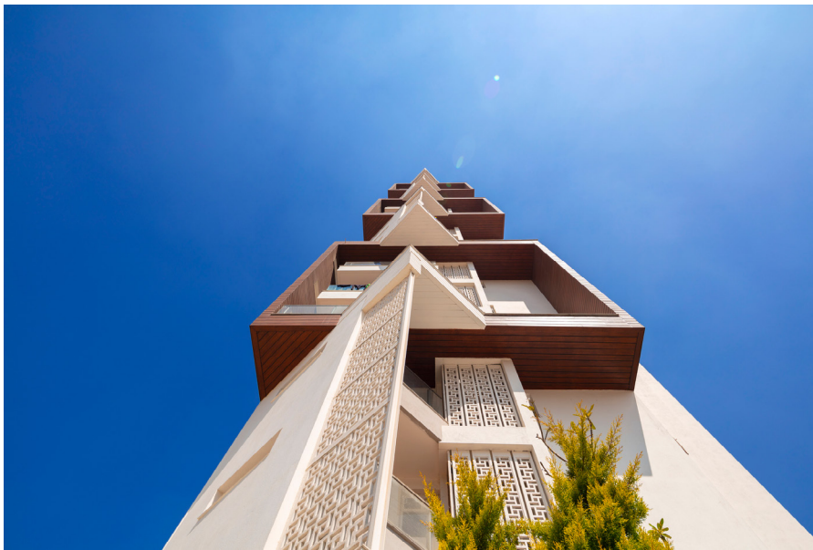
—> Figure 6.10: Balconies and shading elements in the form protects the building from excessive solar gain. Source: archdaily.com
