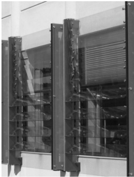
Figure: LRGSS system. The upper glass lamellas are positioned to block the sun gains and the lower ones are redirecting sun illumination deep into the building. Source: Appelfeld & Svendsen, 2013
