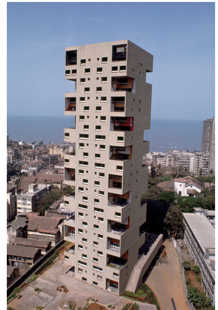
Figure 6.7: Big environment protected opening helps in having effective wind-driven ventilation. Source: http://dome.mit.edu/handle/1721.3/58062
