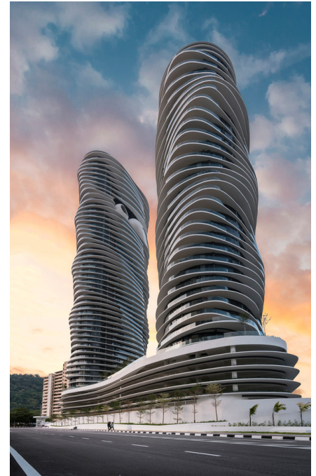
Figure 6.15: Elliptical shape of the building helps in reducing the cooling needs. Source: Archdaily.com
