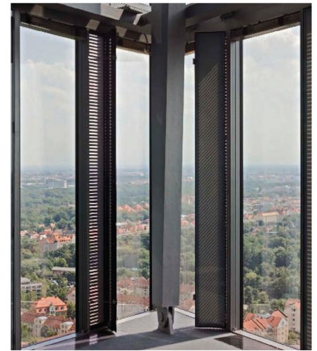
Figure 6.21: The hinged windows and the perforated steel windscreen. Source: (Wood & Salib, 2013).
