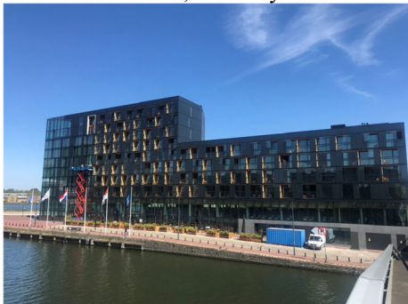
Figure 1: 8-storey hotel Jakarta in Amsterdam made of prefabricated 3D-CLT modules, completed in 2018.
