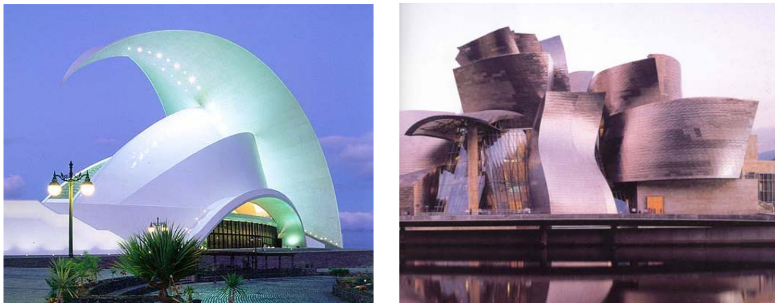
Figure 1.1: It is difficult to predict wind loads on complex building shapes (Internet, [14])
