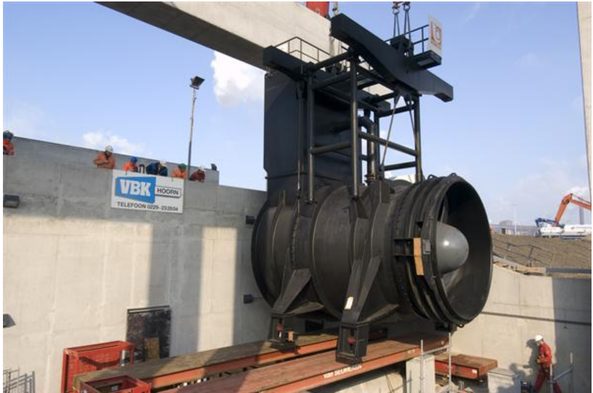
Figure B.1: Proposed horizontal screw pumps
