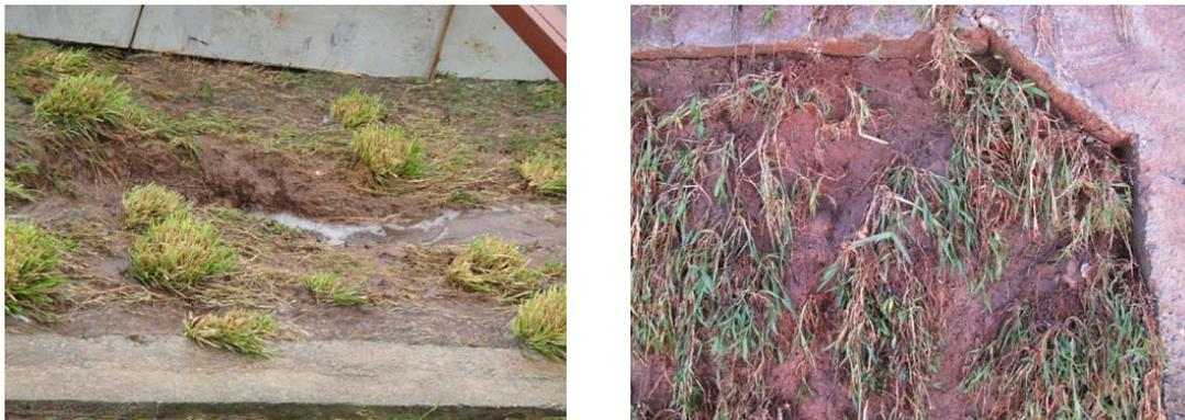
Figure 8: Left: damages amongst Vetiver clumps. Right: poor cover of Bermuda grass and settlement of soil around concrete beams,
