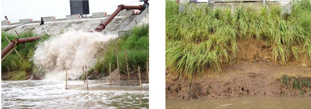
Figure 6: Overtopping flow flying from the berm attacks the dike toe.
