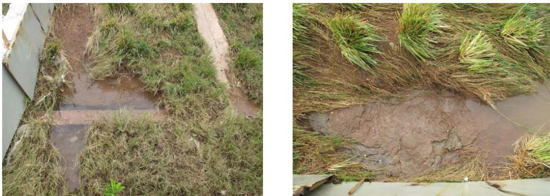
Figure 7: Left: concrete beam was exposed. Right: mortar layer under a top grass sod.
