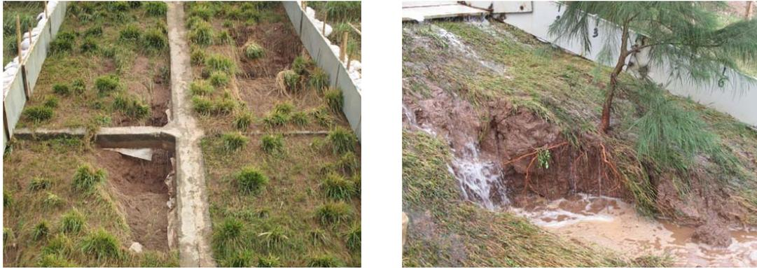
Figure 9: Left: damage around concrete frames. Right: damage extension to the Casuarina tree.
