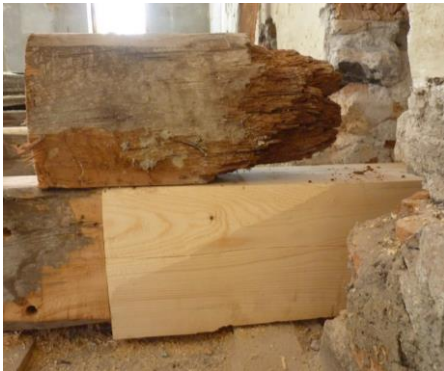
Figure 30: Replacement of rotten wooden beam affected by moisture (Fraunhofer IBP, z.d.)
