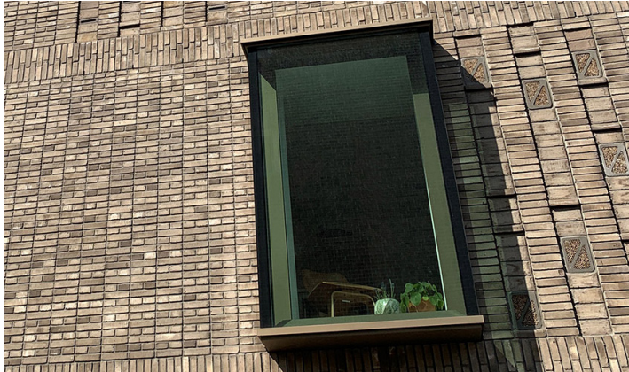
Figure 13: Buro Harro. (n.d.). Façade of the building
