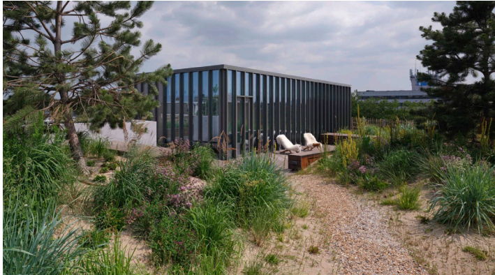
Figure 11: Buro Harro. (n.d.). Roof of the building
