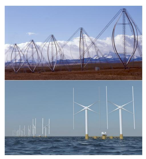
Figure 1.2: Upper: Adecon AL-38 turbines in Pincher Creek, Alberta. Photo by Jos Beurskens (Möllerström et al., 2019). Lower: The NENUPHAR concept of floating VAWT with a double  $2\times5MW$  rotor concept.
