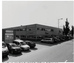
medium sized industrial building; Asterweg
