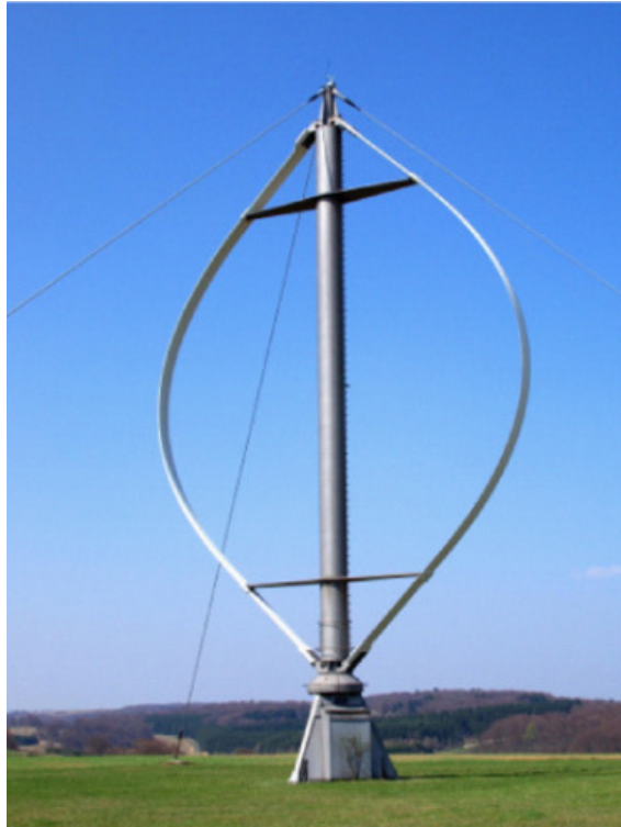
Figure 15: Éole, the world's largest VAWT[130]
