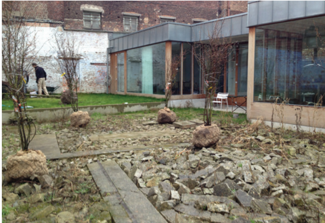
FIGURE 3 Construction of a framework for the different garden zones through differentiated soil treatments. The design of the central garden (bottom half of the picture) literally breaks through the sealed character of the site by scattering the concrete slab into the plant substrate. Several strips of concrete are left unscattered to be used as pathways. The plantings of Amelanchier ovalis ensured the client of the direct presence of structuring green. In the upper garden (top half of the picture), reachable by a concrete step, the concrete slab was fully removed and grass with two Celtis occidentalis was provided. This approach enabled different modalities of floral and human recolonisation and in doing so stimulated a variety of garden experiences. (Photograph by Geert Meysmans, 2013. Reprinted with permission).
