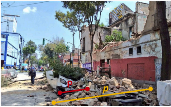
Fig. 6. Example of debris extension evaluation.
