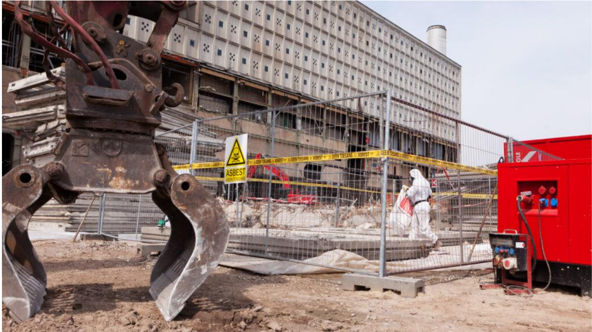
Figure 2. Asbestos remediation at Centrale Harculo [Photograph]. Reprinted with permission from RPS (2018).
