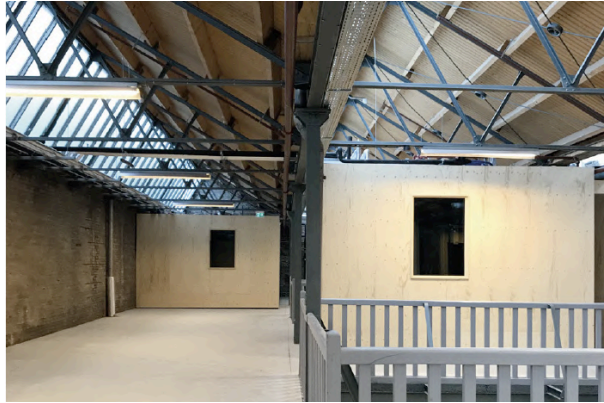
Figure 44: saw-tooth roof (Maurer United Architects, 2020).
