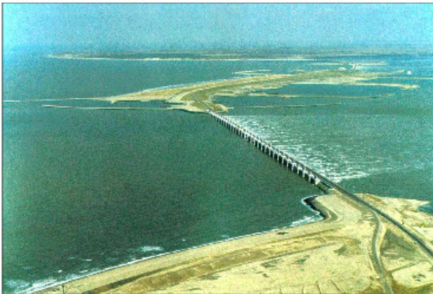
Figure 3.2. Storm-surge barrier under normal conditions (Source: Huib de Vriend, 2004)
