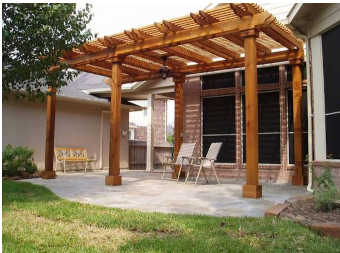
Figure 18: Gazebo with wood shield as bases of the posts
