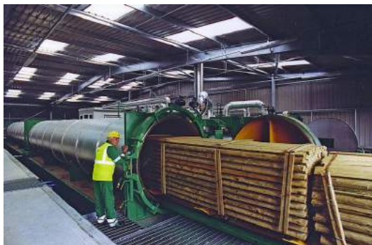
Figure 19: Pressure treatment plant
