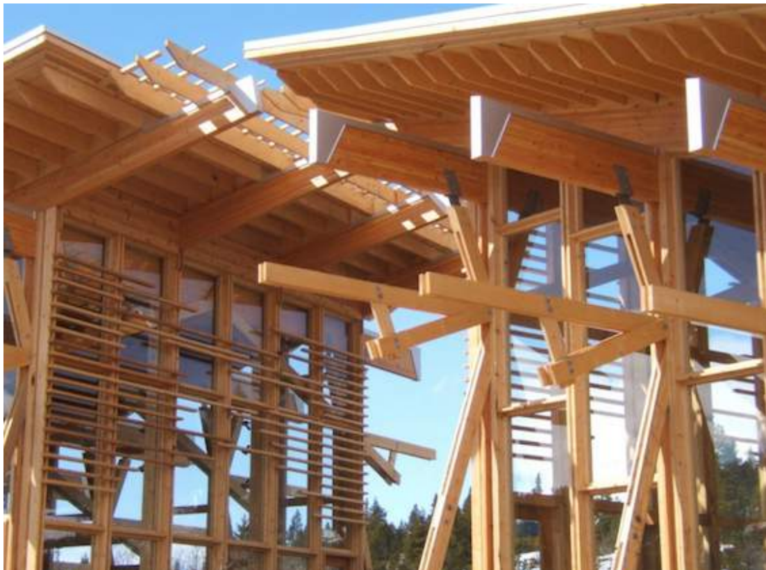
Figure 16: View of the metal flashing solution for Yukon Suspension Bridge by Scott M. Kemp Architects
