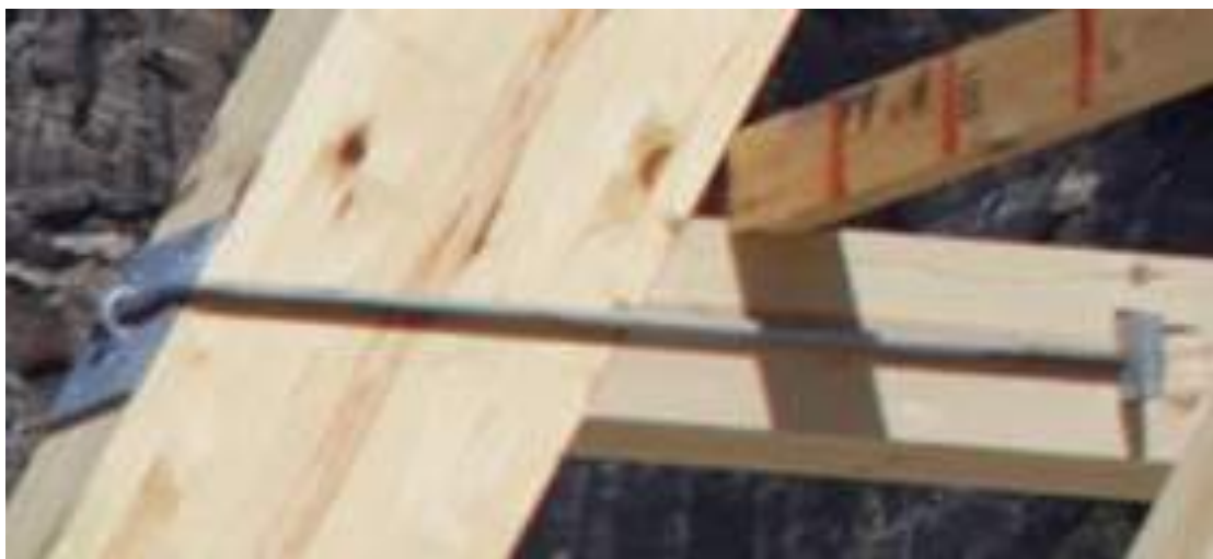
Figure 29: The demountable joint used for the structures of Salt by Rintala Eggertsson Architects
