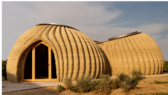
Figure 1.3: 3D-printed house from mud, in which less than 6 kW of energy is consumed for production. ( Iago Corazza, 2021 ).
