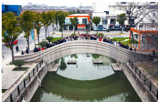
Figure 1.4: 3D-printed bridge in Shanghai, with a length of 26.3 m. ( Ravencroft, 2022 ).
