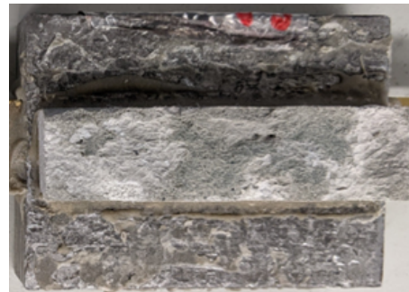
Figure D.18: Top debonded part of Specimen TG20-A-2
