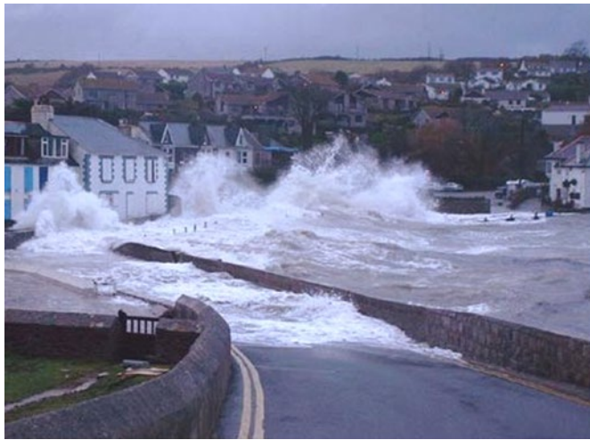
FIGURE 1.1-4: FLOODING CAUSED BY OVERTOPPING. ONLINE IMAGE. RETRIEVED OCTOBER 26 TH 2012 FROM WWW.RESEARCH.PLYMOUTH.AC.UK/CERG/FIELD_OF_WORK/EPIRUS.HTM
