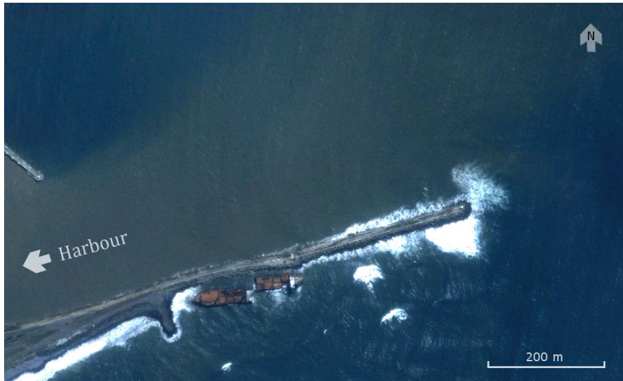
FIGURE 1.1-1: BREAKWATER AT PORT ENTRANCE OF EAST LONDON, SOUTH AFRICA. GOOGLE EARTH. ONLINE IMAGE. RETRIEVED OCTOBER 26TH 2012 FROM GOOGLE EARTH.
