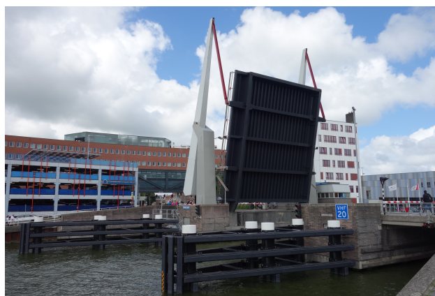
Figure 1.1: Steel-piled fender structure around a movable bridge [3]
