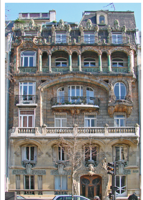
Figure 3: the Lavirotte building, recent photograph 17
