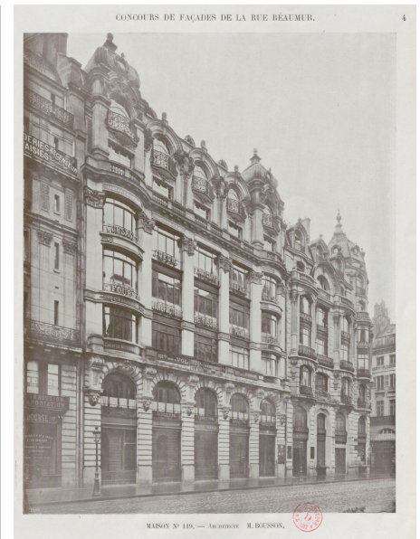
Figure 6: Façade of M. Bousson 20
