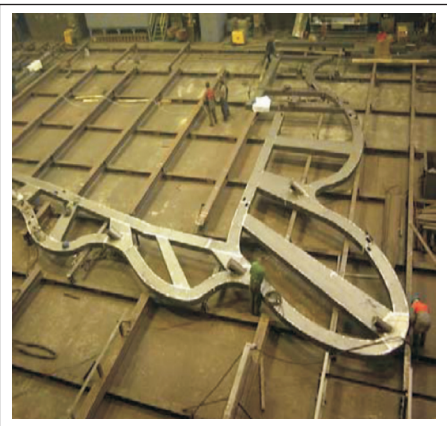
Figure 4.17: Steel plates welded together to form the vierendeel truss
