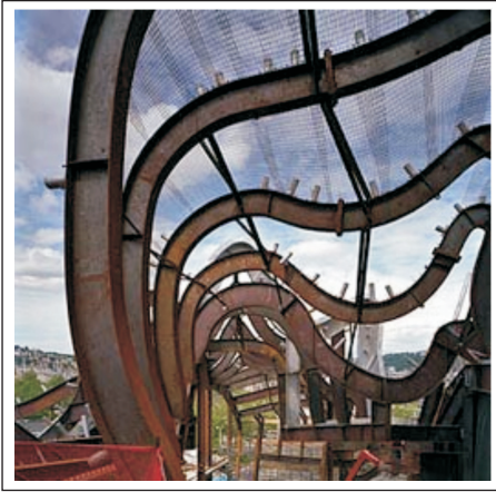
Figure 4.10: The curving steel beams
