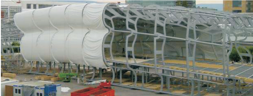
Figure 4.18: PVC-membrane pre-stressed between the steel frames
