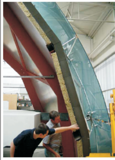
Figure 2.1: The separation of the structure and the skin (Kunsthau, Graz)
