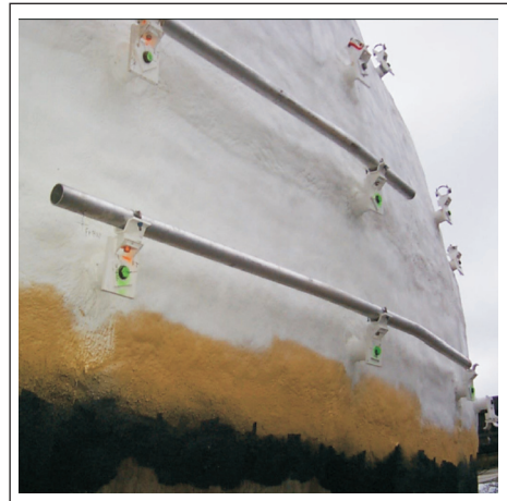
Figure 4.13: The tube system supporting the skin panels
