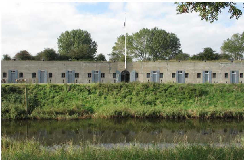
Figure 2.2 Example of a fort of the Stelling van Amsterdam (Fort Vijfhuizen, 1899, situation 2006).
