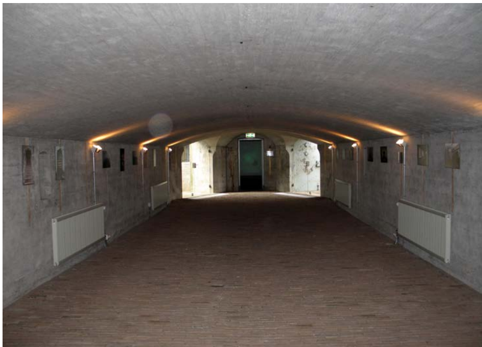
Figure 6.1 Example of a plain concrete vault (Fort near Vijfhuizen, 1899, situation 2006).
