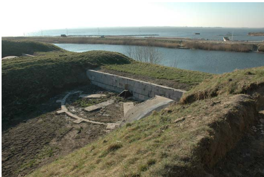
Figure 2.1 Example of the use of plain concrete made with broken bricks in a 19 th century military structure. The wall is rendered and with imitated joints (Fortification Hellevoetsluis, built from 1880 onwards; situation 2012, picture Wido Quist).
