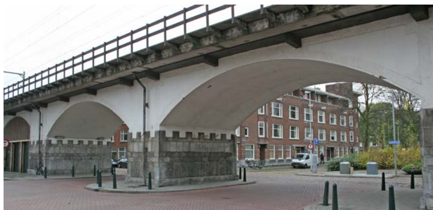
Figure 2.8 The once largest reinforced concrete structure in the Netherlands, the Hofplein railway viaduct in Rotterdam (van Hemert, 1900-1908, situation 2009).
