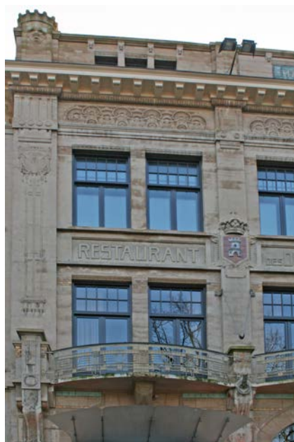
Figure 7.2 Façade of a reinforced concrete building, combined use of artificial stone and kunstzandsteenpleister (artificial sandstone render, former hotel-restaurant “De Twee Steden”, The Hague, Joh. Mutters Jr, 1904-1906, situation 2010).
