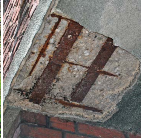
Figure 6.18 Floor construction made with a combination of flat strips and round bars for reinforcement (Housing, The Hague, 1930s, exact year and architect unknown, situation 2009).
