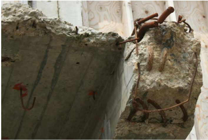
Figure 6.13 Plain circular reinforcement for main reinforcement and stirrups of a beam (Central Station Rotterdam, 1950-1957, S. van Ravesteyn, picture taken during the demolition of the station in 2008).
