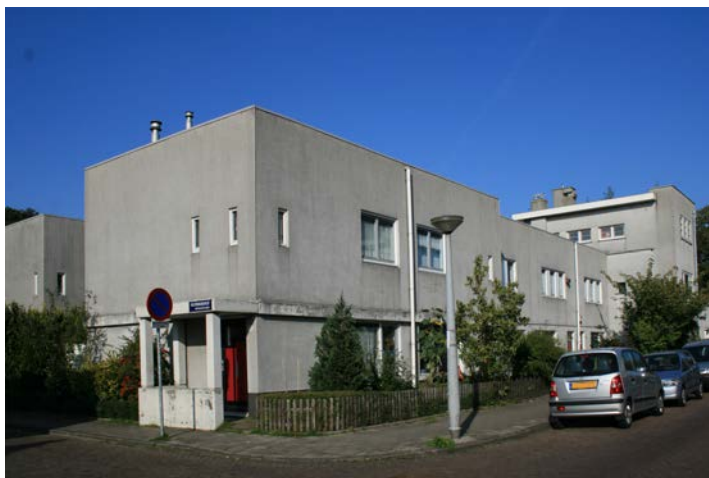
Figure 2.9 Housing made with one of the many building systems used in Betondorp, the Bron system; a three leaf prefabricated reinforced concrete wall made with different concrete types: the outer leaf with gravel as aggregate, the interior and insulating layer with breeze ( sintels ) and in between a breeze filling. The concrete surface was originally brushed but is now plastered (see Kuipers, 1987, p. 191) (Amsterdam, D. Greiner, 1923-1925. Situation 2008).
