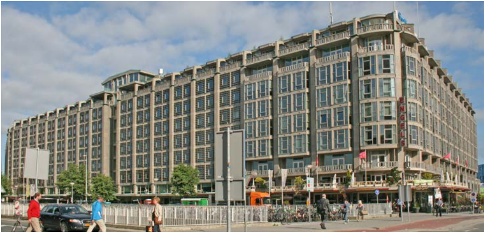
Figure 7.20 The office building Groothandelsgebouw is an example of combining pre-fabrication with different surfaces finishes. The building was painted white to cover up repairs in the 1960s. During large scale restoration works in 2001-2005 the paint was removed; degradation problems are still present (Rotterdam, H. Maaskant & W. van Tijen, 1950).
