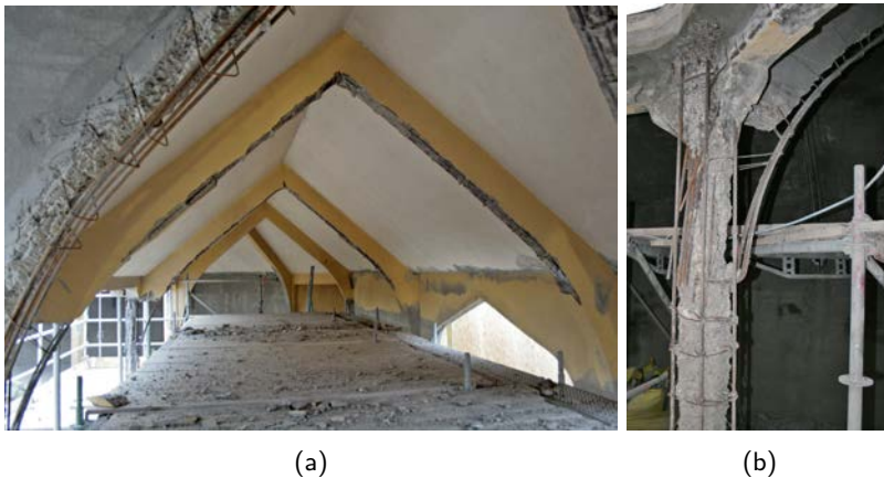
Figure 9.6 Large scale concrete removal with hydrodemolition (circumambulation passageway of the Pilgrimage church in Brielle, H. Goossens (reconstruction), E.J. Margy, 1912, situation 2010). a) Overview of concrete rafters, partial concrete removal. b) Column after removal of the entire original surface and most of the original concrete, exposing the reinforcement.
