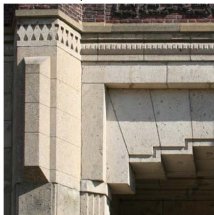
Figure 7.4 The original material of the column and arch is tuff stone, only local replacements were carried out in well-made natural stone imitations (top of the column) (Faculty of Architecture, former Faculty of Chemistry, TU Delft, G. van Drecht, 1918-1923, situation 2011).
