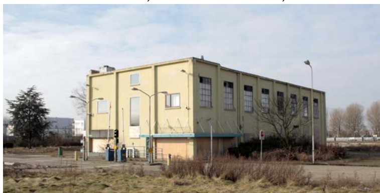
Figure 2.6 Earliest known still remaining factory building in the Netherlands designed according to the Monier system and built by Amsterdamsche Fabriek van Cement-IJzerwerken Wittenburg (Calvé factory, Delft, 1905, situation 2010).
