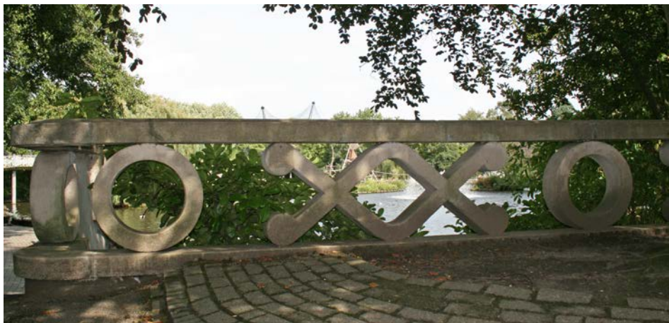
Figure 7.78 Decorative concrete balustrades (Zoo Blijdorp, Rotterdam 1939-1941, situation 2010).
