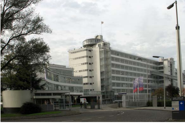
Figure 1.2 Example of the conversion of a former factory into an office building (Van Nelle factory, J.A. Brinkman and L.C. van der Vlugt, 1926-1931, situation 2006).
