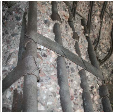
Figure 6.20 Stirrups made from strips in combination with plain reinforcing bars; notice the coupling of the bars above the strips and the annealed wires to connect the elements (emplacement of the Hofplein railway viaduct, Rotterdam, Van Hemert, 1904, situation 2009).
