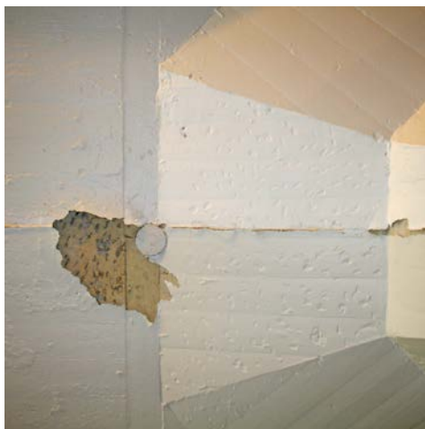
Figure 7.22 Soffit and head of a mushroom column, currently painted, with local detachment of paint. Several, irregularly spread holes in the concrete surface, applied to increase the roughness, indicate that the soffit and column were previously plastered (Van Nelle factory, J.A. Brinkman and L.C. van der Vlugt, 1926-1931, situation 2008).
