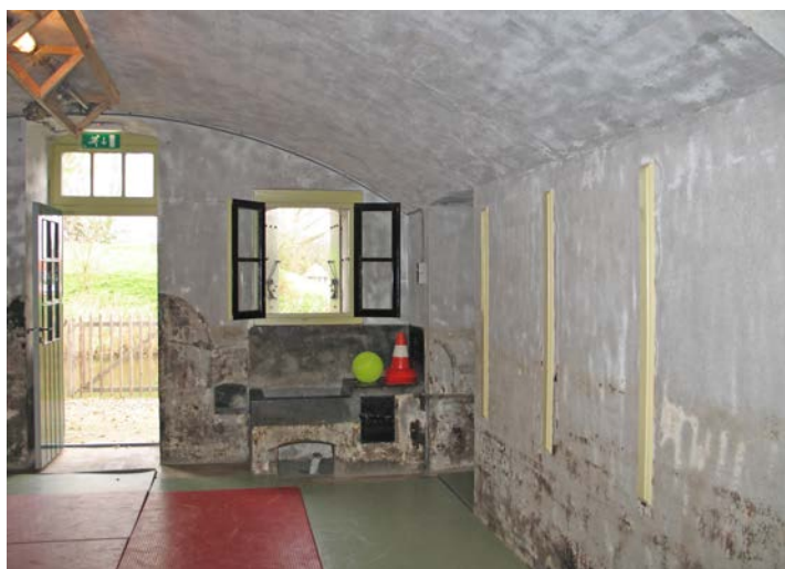
Figure 8.15 Interior of Fort Bezuiden Spaarndam with visible wooden boards cast into the concrete wall for the later attachment of interior elements (situation 2006).
