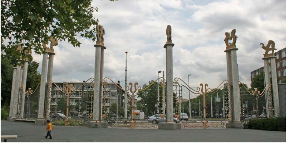
Figure 7.11 Example of use of decorative concrete instead of natural stone for sculptures due to material scarcity (Main entrance Zoo Blijdorp, Rotterdam, S. van Ravesteyn, sculptures L. Bolle, 1939-1941).
