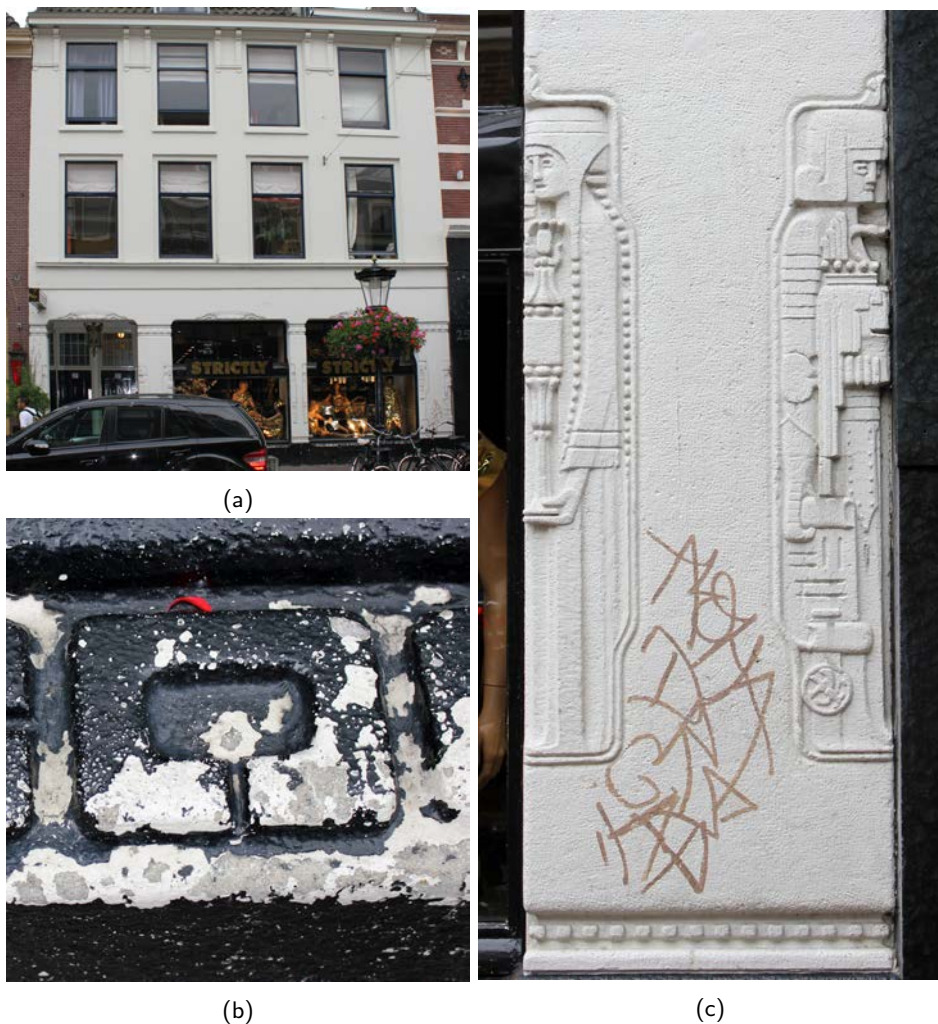
Figure 7.62 Example of the use of a specially carved timber formwork for reliefs in concrete for the refurbishment of a shop façade (G. Rietveld, Utrecht, Oudkerkhof, 1919, situation 2011). a) Overview with the refurbished ground floor. b) Where the paint has chipped off the use of concrete can be identified. c) Detail of a column with reliefs. The surface has been tooled, and in the meanwhile painted white, easily leading to the assumption that natural stone had been used.
