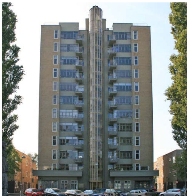
Figure 2.10 The first high-rise housing project in the Netherlands, the “Wolkenkrabber”, was made with a reinforced concrete structure (Amsterdam, J. F. Staal, 1932, situation 2009).
