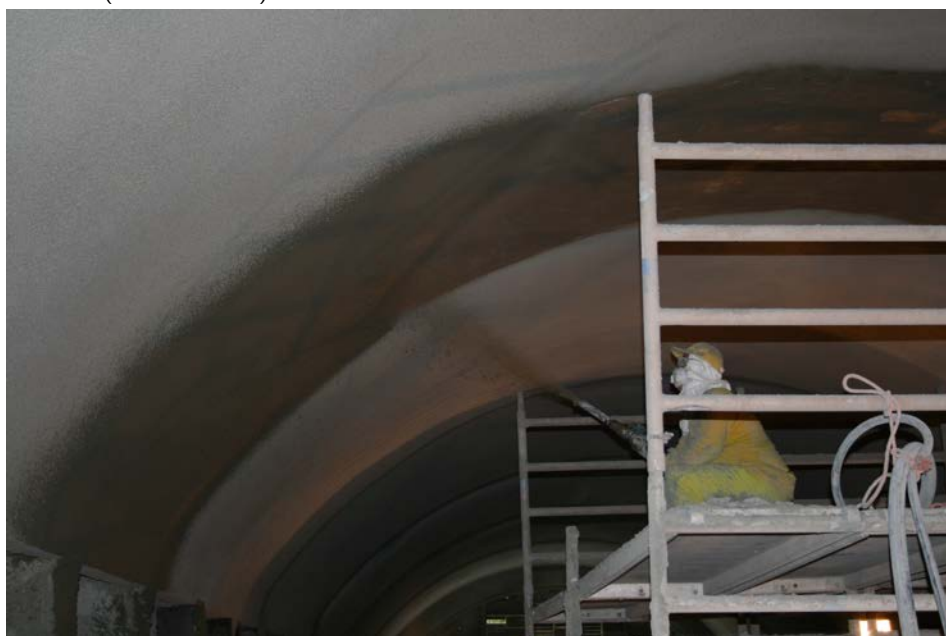
Figure 8.22 Application of sprayed concrete in the vaults of the emplacement, this technique was chosen due to the size of the intervention and the costs (Hofplein railway viaduct 1900-1908, situation 2009).
