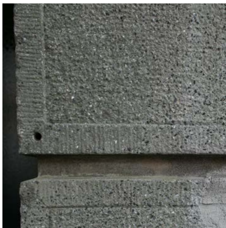
Figure 7.31 Example of a bush hammered surface with chiselled margins; the concrete is made with diabase as aggregate (housing, 1930s, exact date and architect unknown, Rotterdam).
