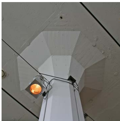
Figure 7.53 Geometric pattern based on the technical solution for a timber formwork of a mushroom floor (Van Nelle factory, J.A. Brinkman and L.C. van der Vlugt, 1926-1931, situation 2008, surface originally plastered, now painted).
