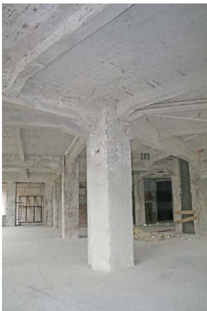
Figure 7.1 Example of the “romantic and brute industrial atmosphere” of the interior of concrete buildings ( Lichttoren , Philips building ED, Eindhoven; Bureau TABROS1920/21, situation during intervention 2007).
