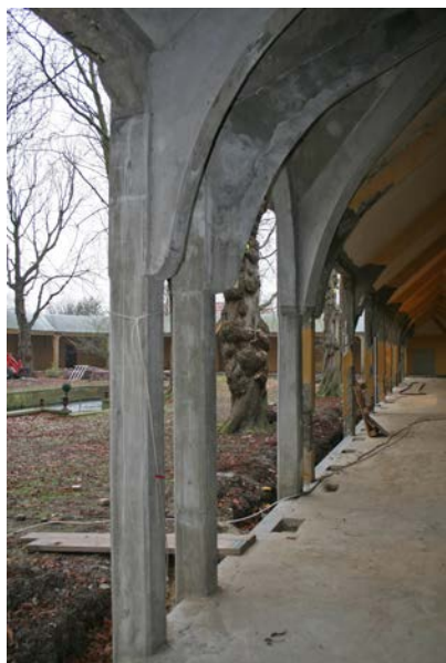
Figure 9.7 Trial repair of three columns to test the workability (sprayed and poured polymer modified repair mortar) and quality of the surface finish (circumambulation passageway of the Pilgrimage church in Brielle, H. Goossens (reconstruction), E.J. Margy, 1912, situation 2010).
