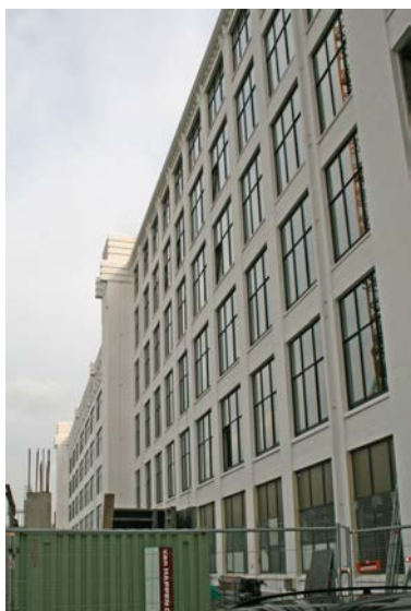
Figure 2.4 Former factory building for Philips Gloeilampenfabriek N. V. (Eindhoven, front part, 1909-1911, A. Beltman, in the back the “Lichttoren” 1920/21, Bureau TABROS; situation 2007).
