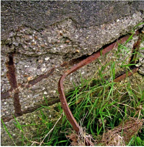
Figure 6.17 Example of an unusual use of only rectangular reinforcement (bomb shelter near Fort Benoorden Spaarndam, 1916 - 1919, situation 2006, picture by T. G. Nijland).
