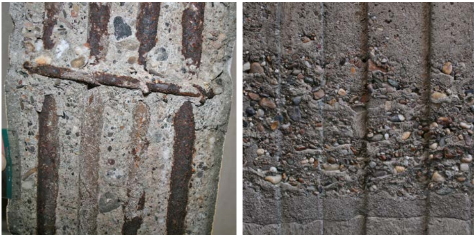
Figure 4.5 Early example of reinforced concrete made with gravel; notice that between the reinforcement bars only smaller sized aggregates are present (circumambulation passageway, Pilgrimage church, Brielle, 1912, situation 2010).
