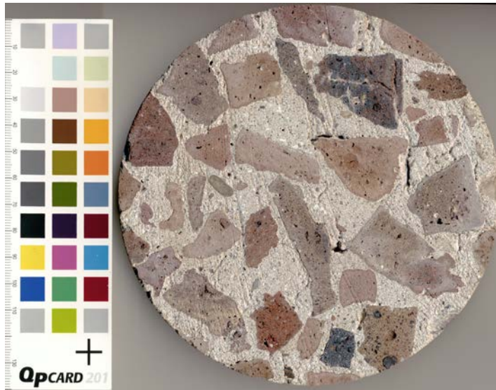
Figure 4.9 Example of plain concrete from the Nieuwe Hollands Waterlinie, ca. 1850 made with broken bricks and a trass-lime binder. The angular shape of the aggregates in combination with manual compaction explains the presence of voids near the aggregates. No contaminations were found along the edges of the aggregate, indicating the use of new bricks and not debris (see also Heinemann et al., 2012) .
