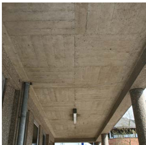
Figure 7.54 Soffit with pattern consciously chosen by arranging individual timber boards perpendicular in squares (Train station Zutphen, H.G.J. Schelling, 1952, situation 2009).
