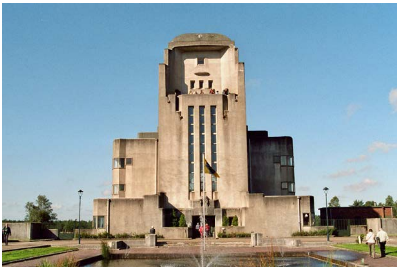
Figure 1.7 Former radio station Kootwijk (J. M. Luthmann, J. Emmen, 1921-22, situation 2006).
