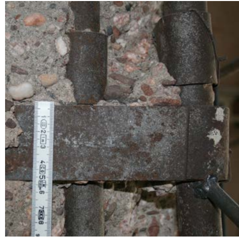
Figure 6.41 Example of a coupling of vertical reinforcement bars above a horizontal stirrups made with strips (emplacement of the Hofplein railway viaduct, Rotterdam, 1904, situation 2009).
