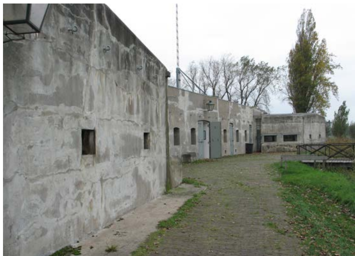
Figure 8.14 Overview gorge façade Fort Bezuiden Spaarndam (1897-1901, situation 2006).
