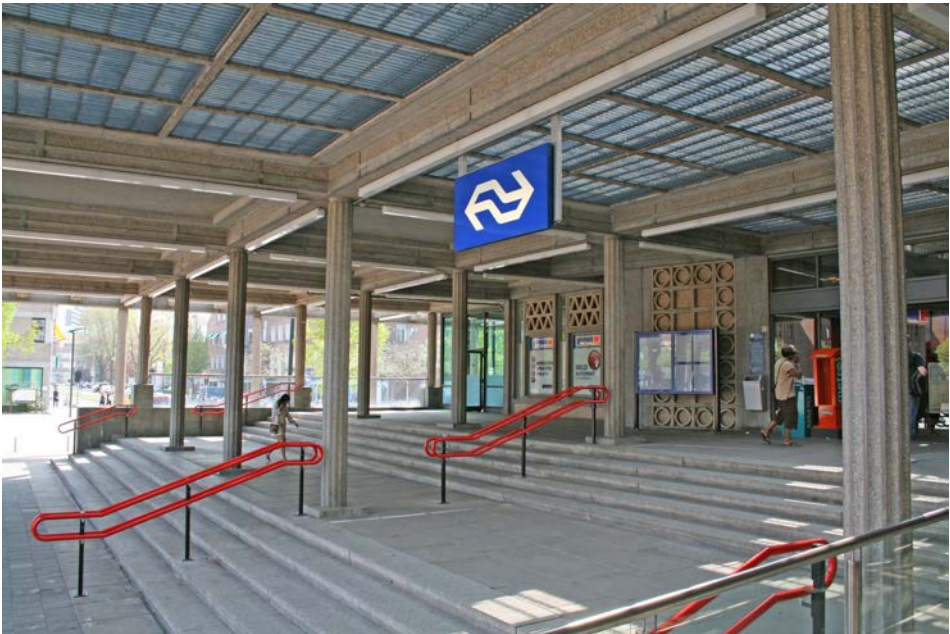
Figure 7.12 Overview of the Railway station Enschede; the beams were made with permanent formwork (Schokbeton) due to timber scarcity after the Second World War (H.G.J. Schelling, 1950, situation 2009, see also Figure 6.45).
