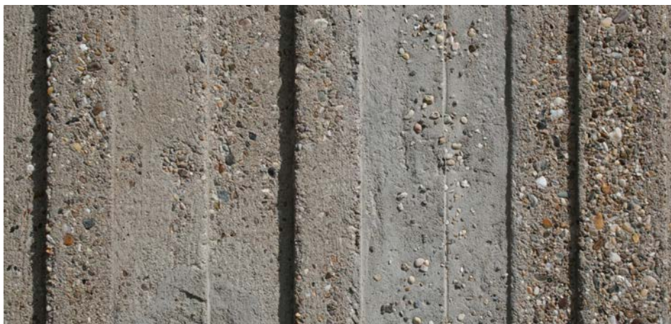
Figure 9.11 Repair of an exposed concrete surface made with blast furnace slag cement and gravel, originally with a wood grain structure. Although several try-outs were made, locally the patch repair can still be distinguished due to the lighter colour and irregularly pressed-in aggregates. The wood grain texture was not reconstructed (Pumping station Parksluizen, Rotterdam; G. J. van der Grinten, 1967, situation 2010).
