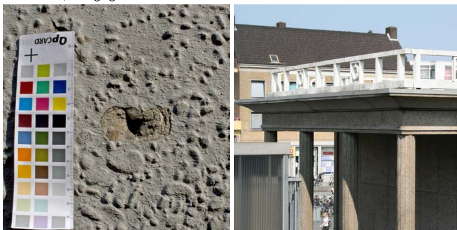
Figure 9.20 Example of a grey painted, previously exposed, concrete surface; the original more brownish colour and colour variations due to visible aggregates cannot be experienced anymore (Olympic stadium, Amsterdam, J. Wils, 1928, situation 2008).
