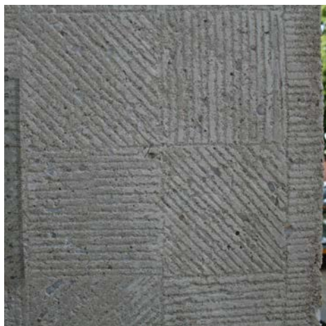
Figure 7.34 Example of horizontal, vertical and diagonal tooling with chiselled margins of prefabricated concrete elements ( Paleis van Justitie , Arnhem, F. Sevenhuysen Jr., 1953-1963, situation 2010).
