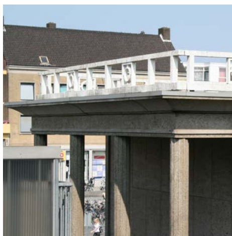
Figure 9.21 Example of the colour change caused by surface treatments: the original composition of the prefabricated balustrades is white Portland cement with Rhine gravel, claustra in the middle of the balustrade made with white gravel and sand blasted (Schelling, 1952b); the architect explicitly rejected painting of concrete (Train station Hengelo, H.G.J. Schelling, 1952, situation 2009).
